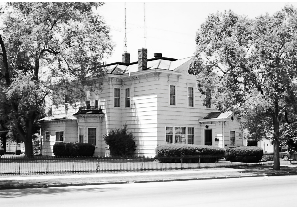
The house-in-town seen from Main Street
